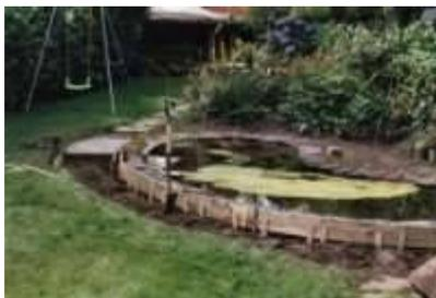
Gravel boarding going in around the pond edge: this is the area where the ground level needed to be raised. ([View bigger image.](#))
