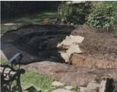
***Here you can see the liner underlay and, underneath that, the loft insulation that I used for cushioning.***
