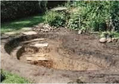
***Pond hole: the foreground shows where the earth was built up to cope with the slope in the garden.***
